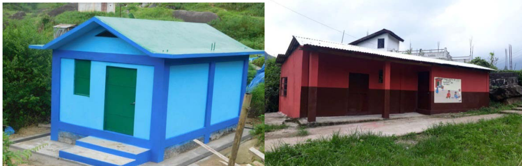
Community Storage Shed for Non-Biodegradable Wastes
