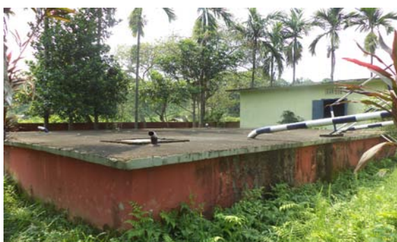
Clear Water Reservoir
