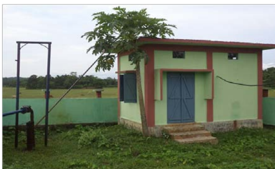
Bore well and Pump House
