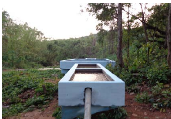
Pre-Sedimentation Tank & Slow Sand Filter
