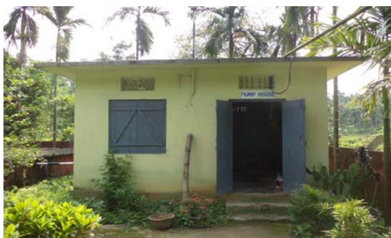
Bore well and Pump House
