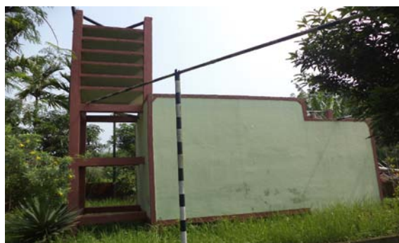
Iron Removal Plant
