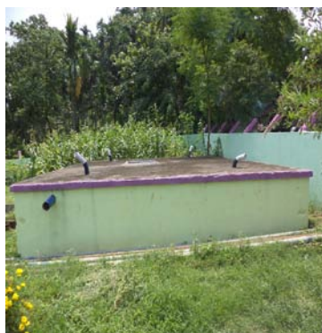
Clear Water Reservoir
