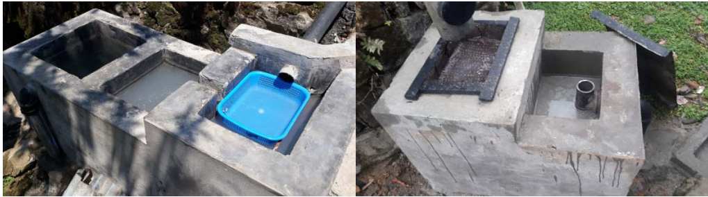
Household Wastewater Oil Trap cum Soakpits
