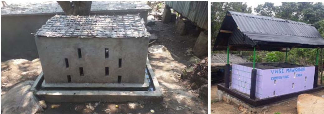
Household Wastewater Oil Trap cum Soakpits
