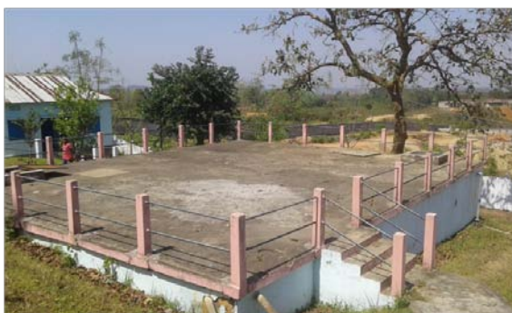
Clear Water Reservoir
