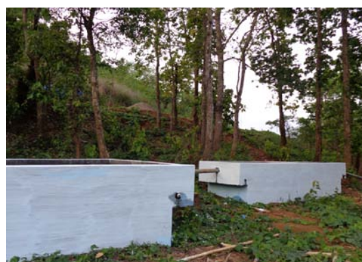
Pre-Sedimentation Tank & Slow Sand Filter
